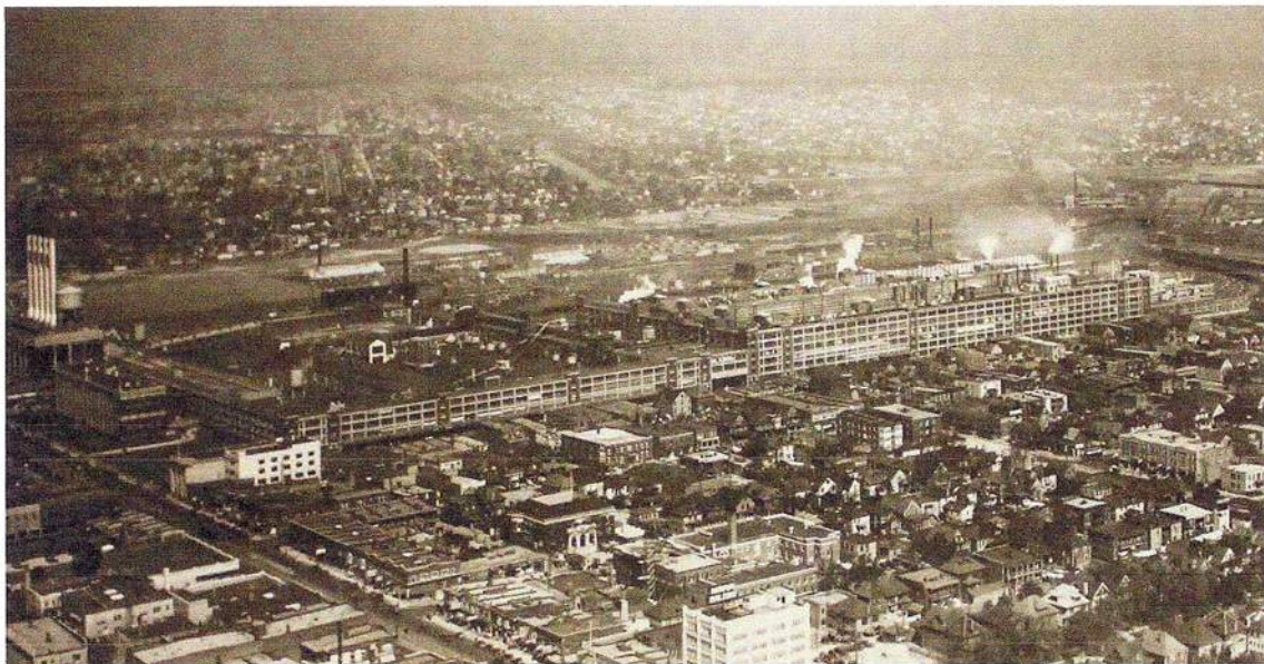
Figure 2: Ford Highland Park Plant 1927, looking northeast; Manchester Street façade in center. (Source: Benson Ford Research Center, Acc 1660, Box 130).
